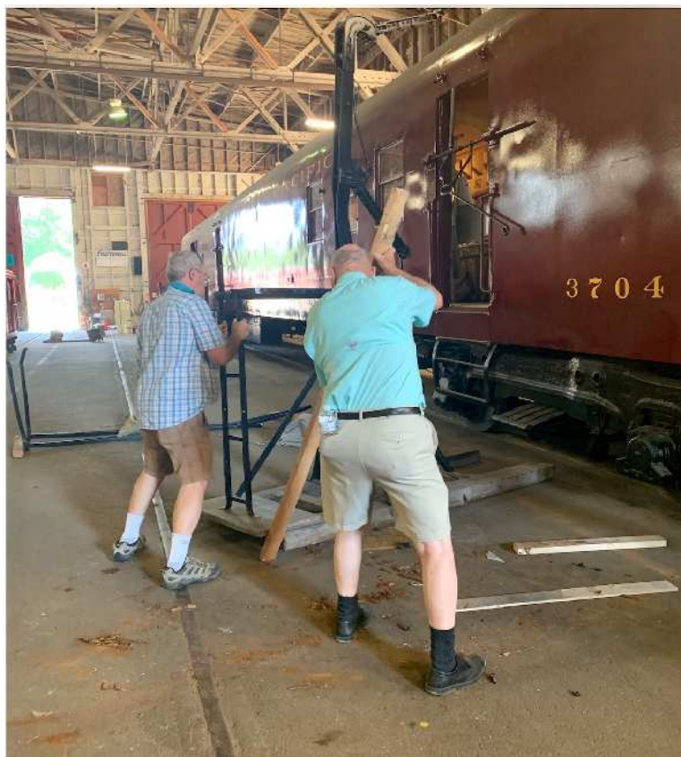
John Cornish & Fred Dannels (Canad Post retirees) moving the 'catch post' into position
