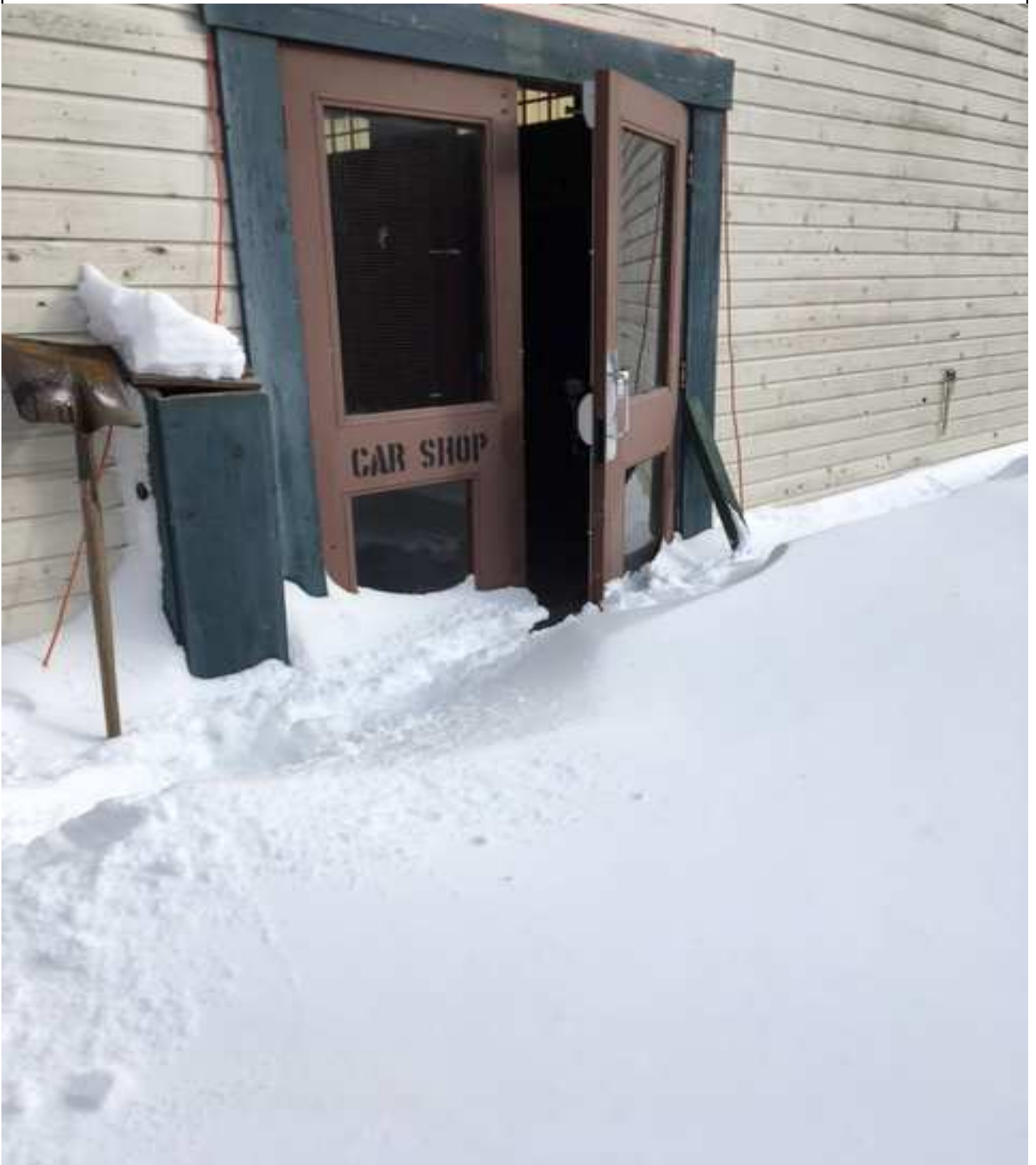
This photo by Gordon Bell shows that on some days we actually had to shovel our way to doors in order to be able to access our buildings as in this scene of getting into the PGE Shop!
